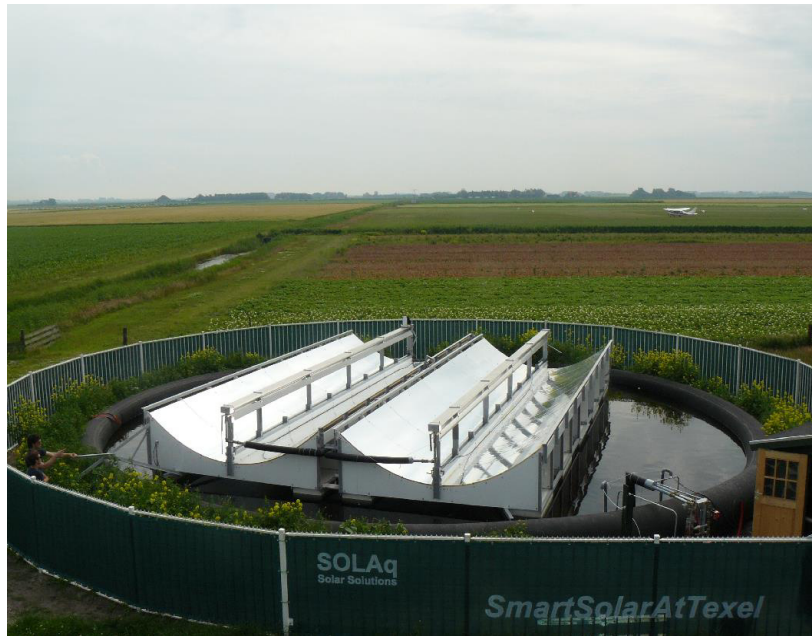
Fig.8. Floating parabolic trough mirror field in an artificial pond at Texel, The Netherlands.
